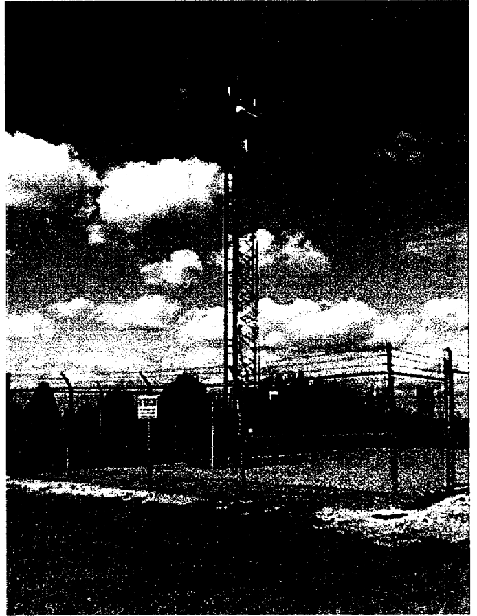
Pictured is the Secondary Meteorological Tower. This station obtains measurements at a height of 10 meters, and provides backup data for the Primary Meteorological Tower readings at 10, 60 and 90 meters.
