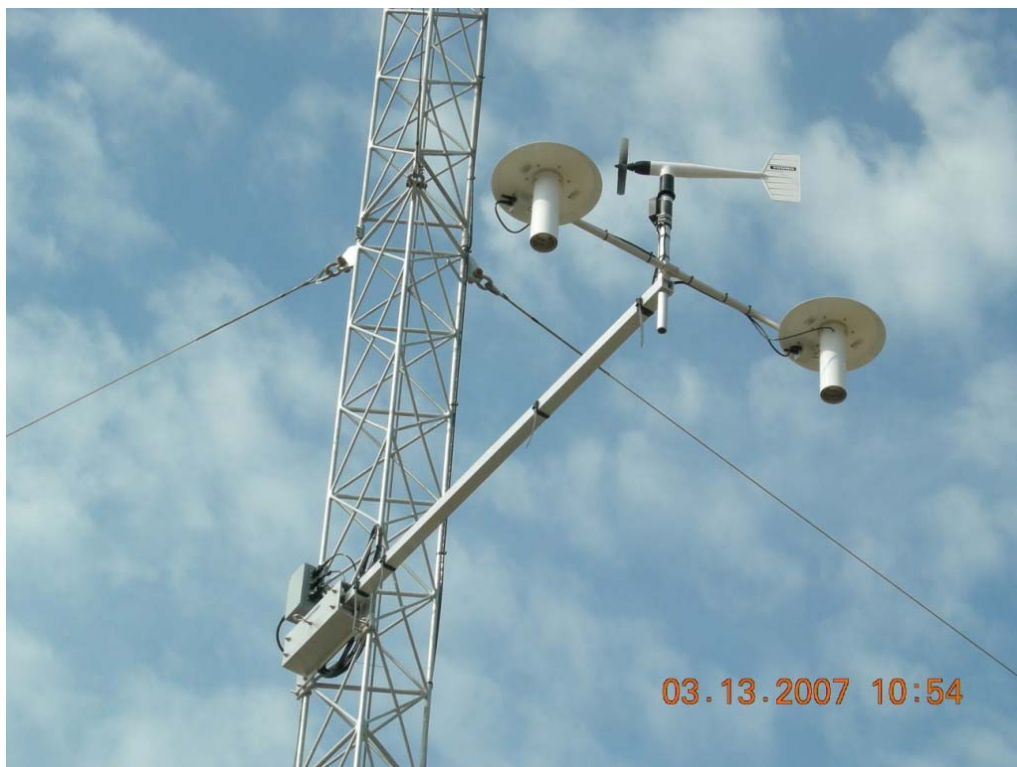
Photo 4 – Lower Level Wind and Temperature Sensors
